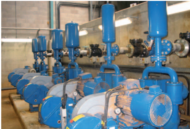
CM piston membrane pumps in a water treatment works in Northern Ireland
